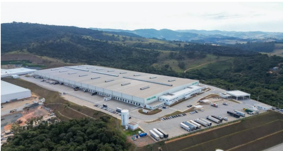
Extrema Business Park, Bloco I – Extrema, MG
