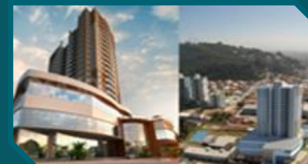
Le Havre Residence
