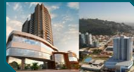
Le Havre Residence
