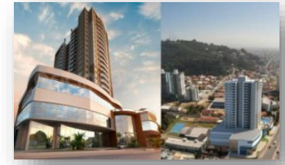
Le Havre Residence
