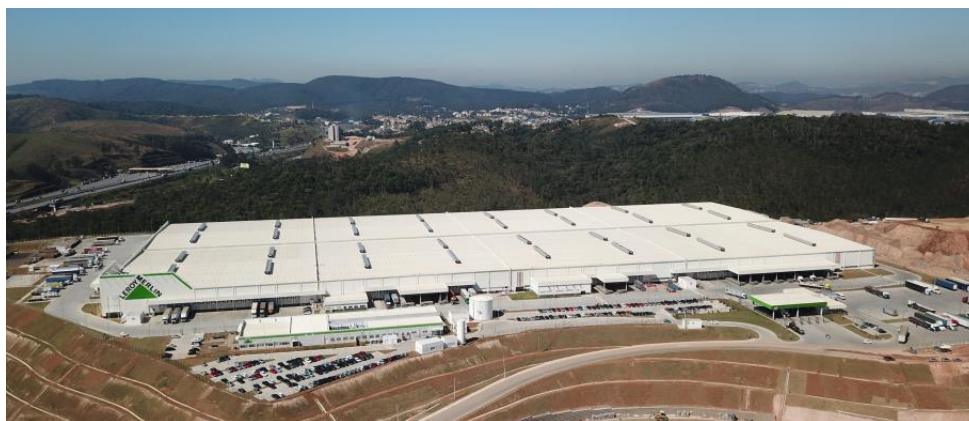
Galpão Leroy Merlin – Cajamar/SP
