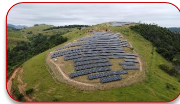
Carmo RBE Light - RJ 5.3 MWp
