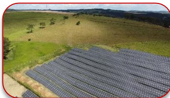
Pains Cemig - MG 3,7 MWp
