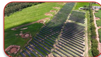
Soleil Copel - PR 3.4 MWp
