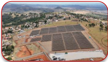
Matozinhos II Cemig - MG 3.3 MWp
