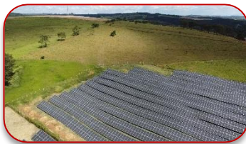
Pains Cemig - MG 3.7 MWp
