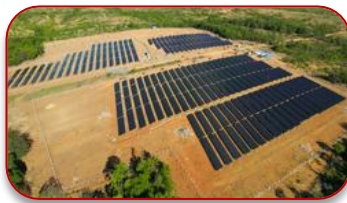
San Remo I & II Cemig - MG 4.8 MWp
