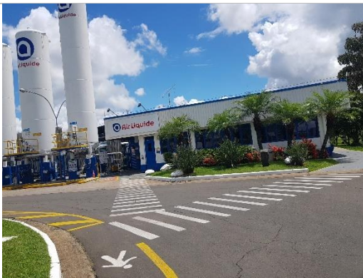
Fachada do bloco principal
