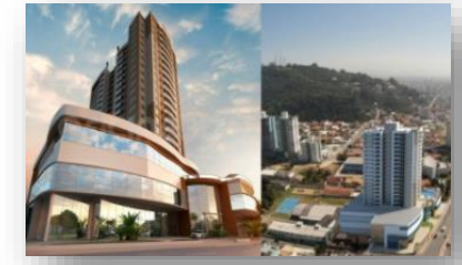
Le Havre Residence
