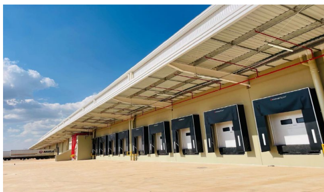
Docas com Dock-shelter Módulo 5 – BTS Libbs.
