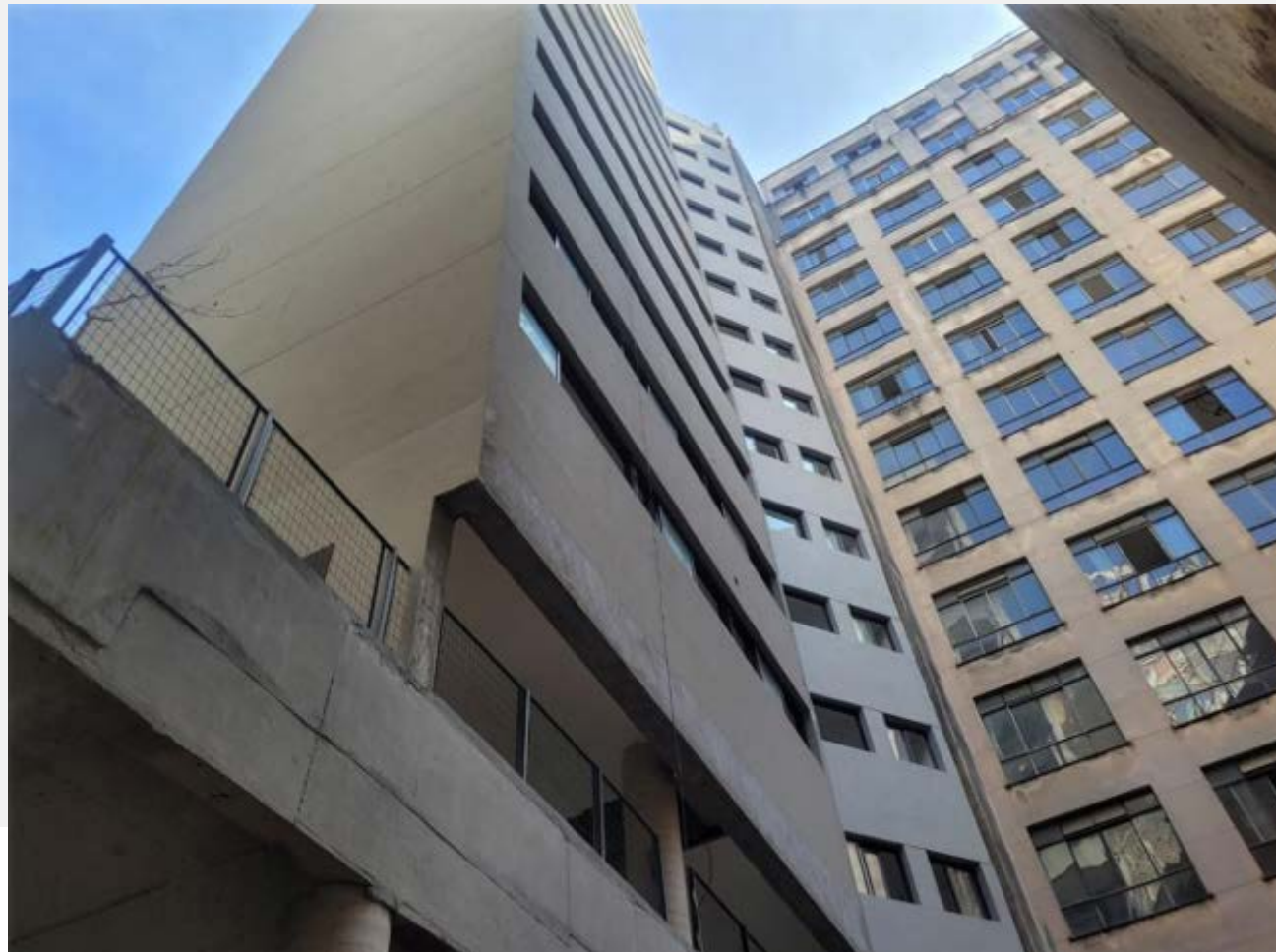
Fachada Bloco C (nov/25)
