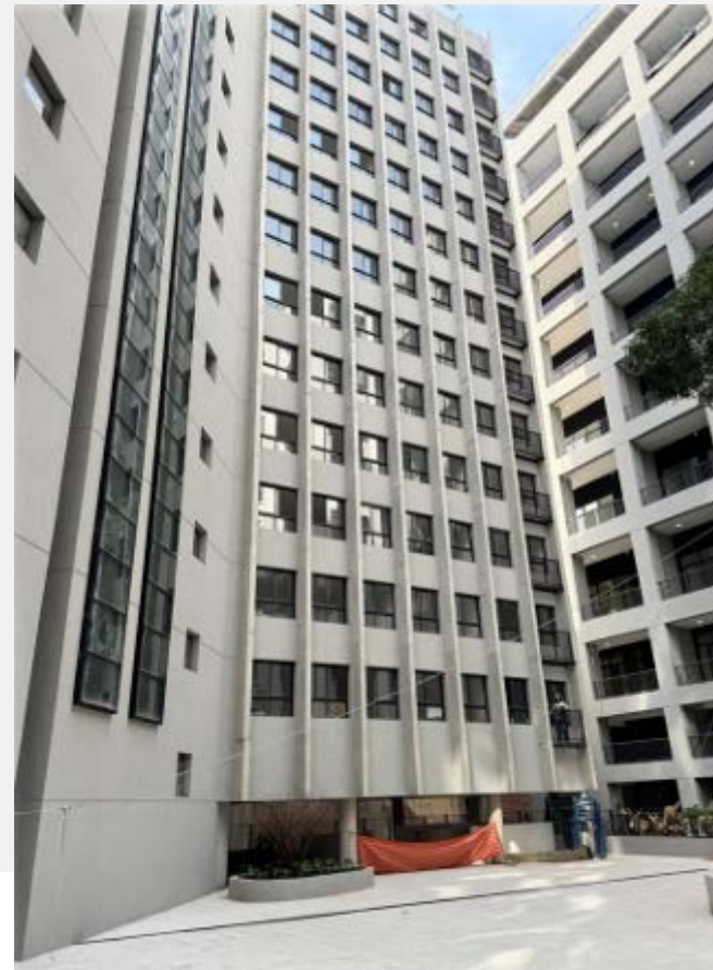
Fachada Bloco C (nov/25)
