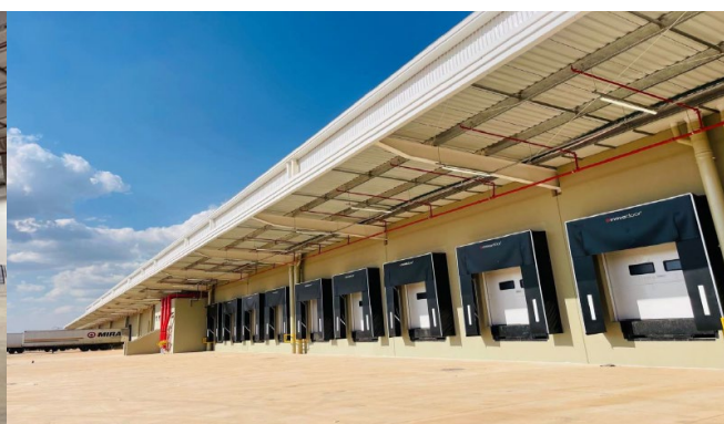
Docas com Dock-shelter Módulo 5 – BTS Libbs.
